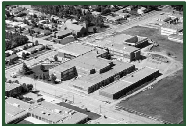
LCI during the construction of the small gym - 1965
